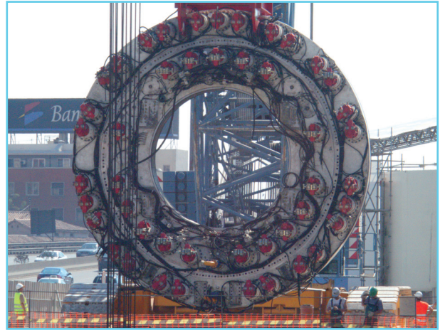
Photo 4. The outer wheel has 50 motors, 29 on the outside face and 21 on the inside face
