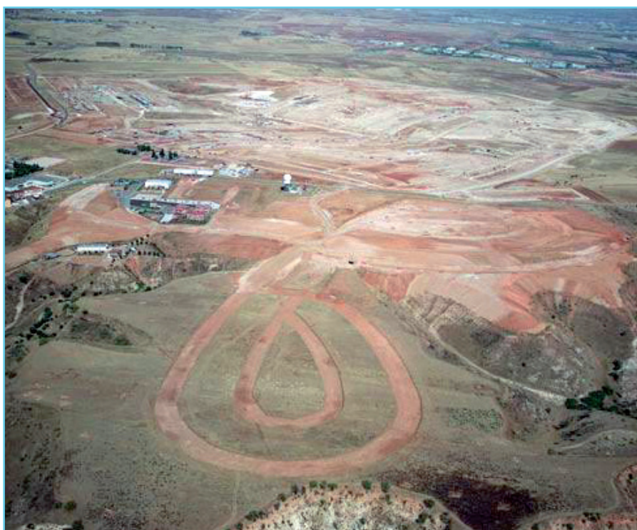
Photo 6. Aerial view of lime stabilized area
