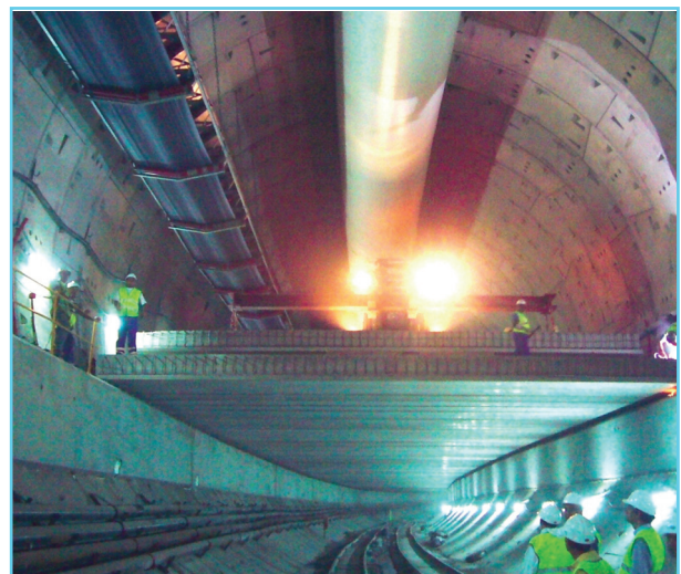
Photo 7. Laying of prefabricated slab
