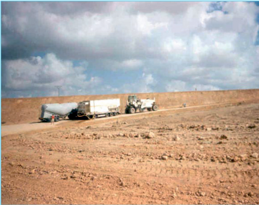
Photo 5. Lime stabilization treatment
