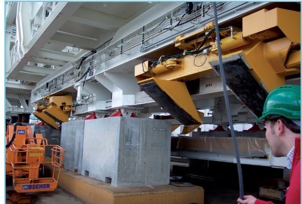
Photo 2. First trailer, with fixed and mobile supports
