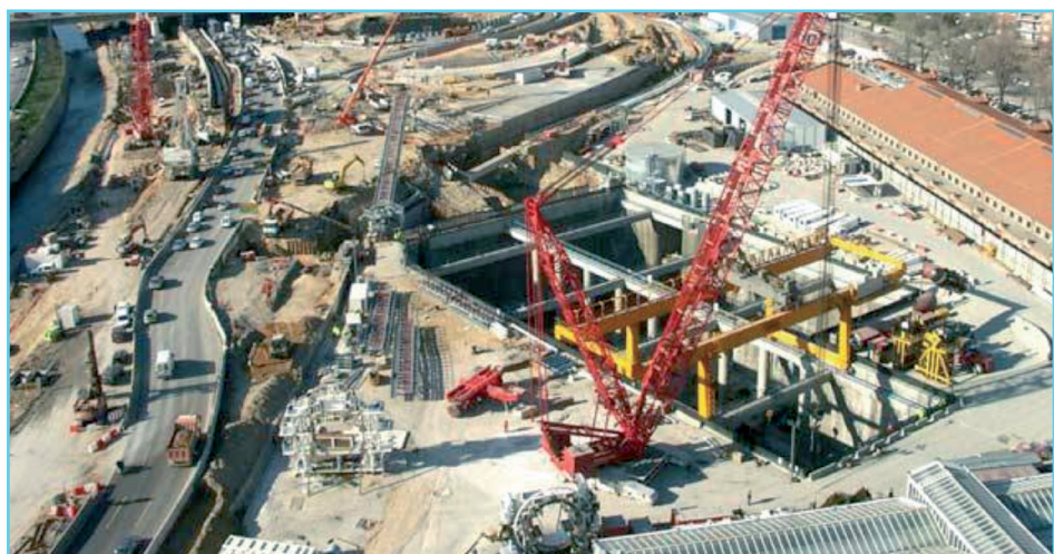
Photo 3. Launch shaft of the South tunnel
