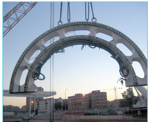
Photo 5. Ring bearing, formed by two parts that support the shield sections
