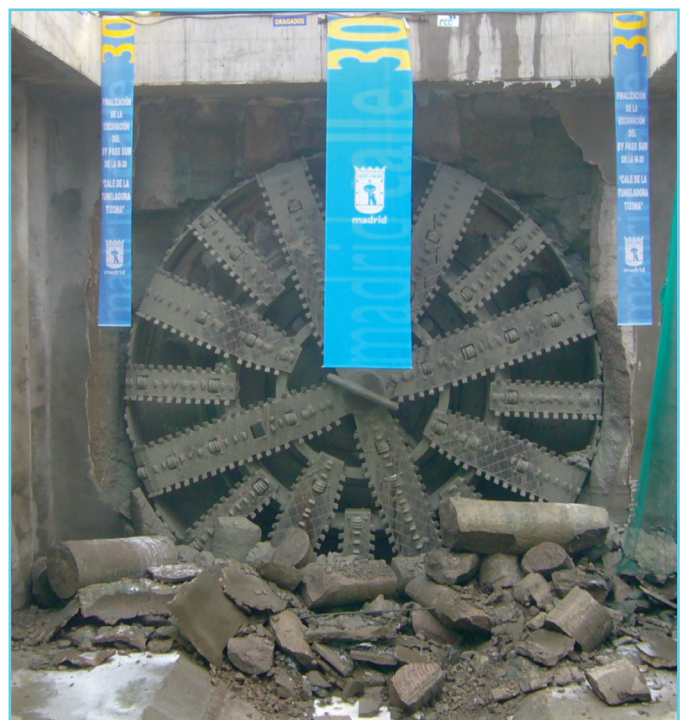
Photo 4. Breakthrough of the South tunnel
