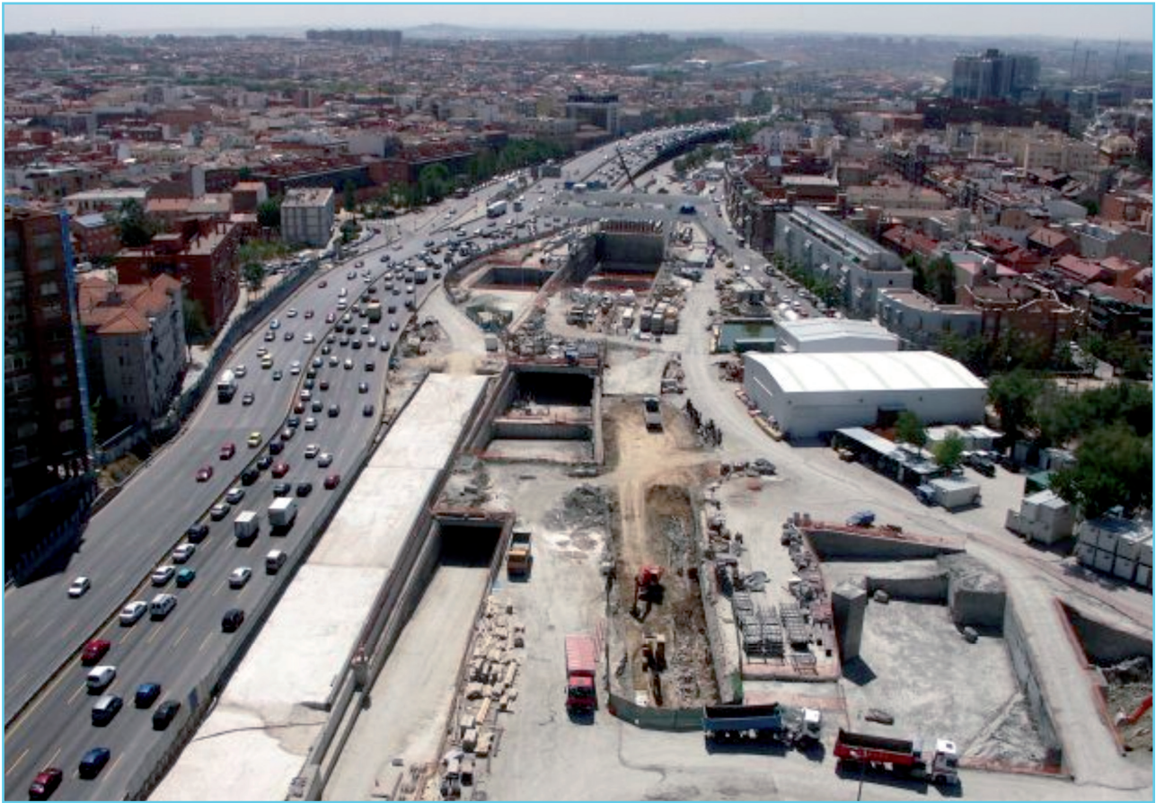
Photo 7. View of launch shaft and surroundings
