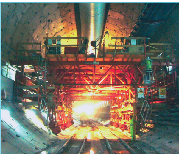
Photo 6. Formwork for the construction of cantilevered supports
