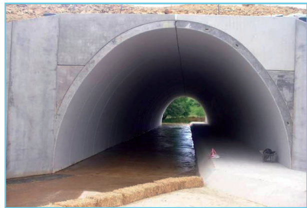
Photo 3. Extended vaulted culvert with pavement for passage of reptiles and amphibians.
