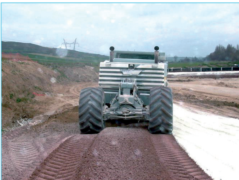
Photo 4: On mixing lime with clay soils, the water content and geotechnical properties of the soil are modified, with an ensuing improvement in its workability and water resistance.
