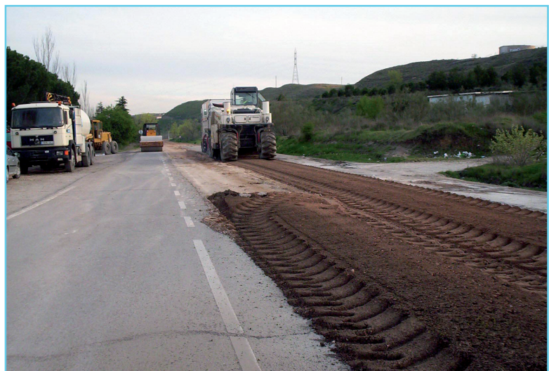
Photo 3. Preparation of soil for lime stabilization during road widening.
